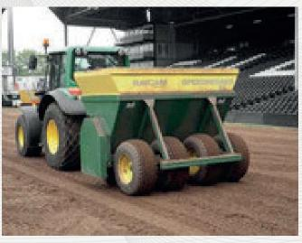
**Loksand**® is a traditional sand and sand based substrate blended with polypropylene fibres. During the mixing process the crimped polypropylene fibres are entwined with the sand increasing the sand's overall strength and resistance.
